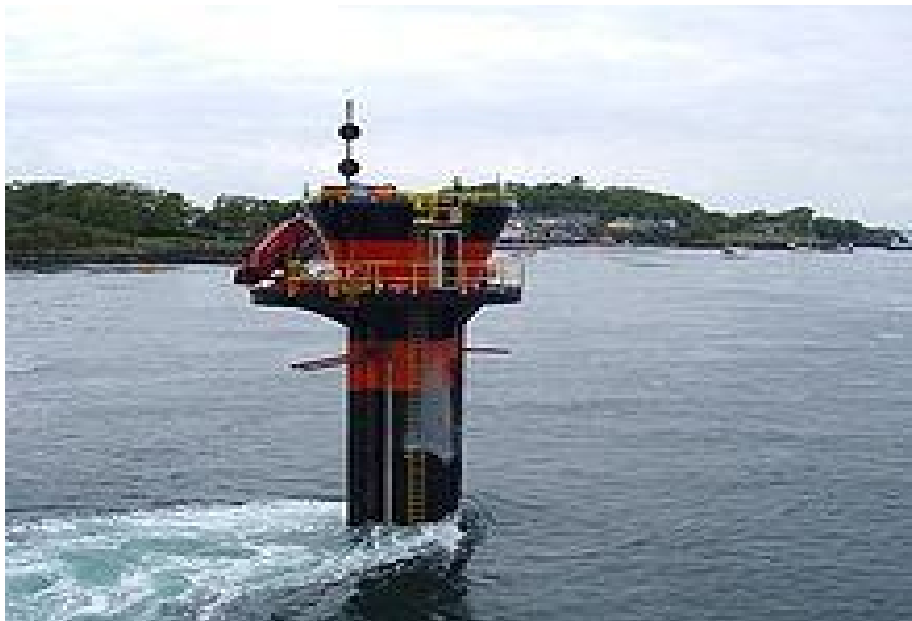
Figure: The world's first commercial-scale and grid-connected tidal stream generator – SeaGen – in Strangford Lough. The strong wake shows the power in the tidal current.
